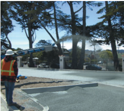
The subgrade consisted of compacted sand with geo-textile, along with three inches of #57 rock and one to two inches of #8 rock.
