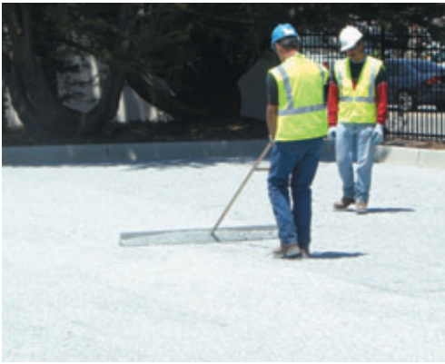
The subgrade consisted of compacted sand with geo-textile, along with three inches of #57 rock and one to two inches of #8 rock.
