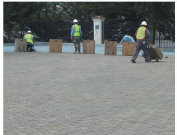
Completed in 2007, neither the contractor nor the manufacturer has received any warranty-related call backs.
