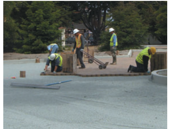
A 7-8 man crew completed the job in just over 1,200 man hours. Weather conditions during the install were dry with temperatures averaging 60 to 70 degrees.
