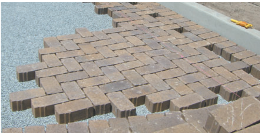
Here, installers have initiated the straight herringbone pattern with a soldier course edging.
